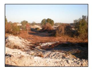
Drainage ditch used to dewater clay-filled areas
