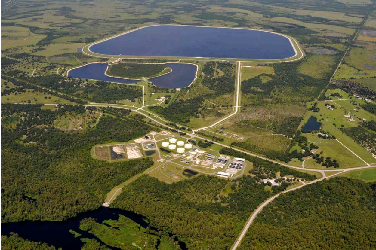
Figure 7.1 August 2010 aerial showing the side channel of the Peace River near S.R. 769 on which the Facility's intake is located, the expanded Treatment Facility, and both the original 0.625 and newer 6.0 billion gallon surface reservoirs.
