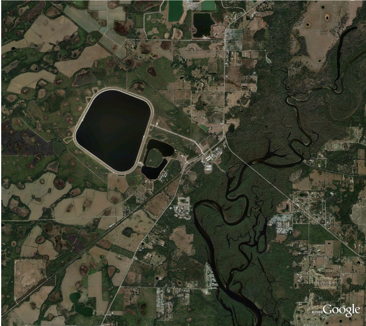
Figure 3.377 Peace River Facility showing site of withdrawal on a side branch of the river, the expanded treatment facility, and both the original 0.625 and newer 6.0 billion gallon surface reservoirs.
